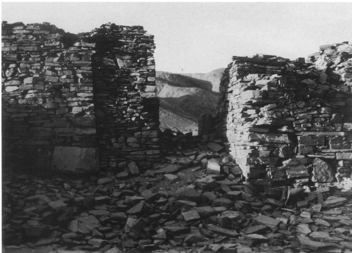
1. The interior of the gate to the praesidium at el-Zerkah. Note how later construction has decreased the width of the opening (p. 168)
