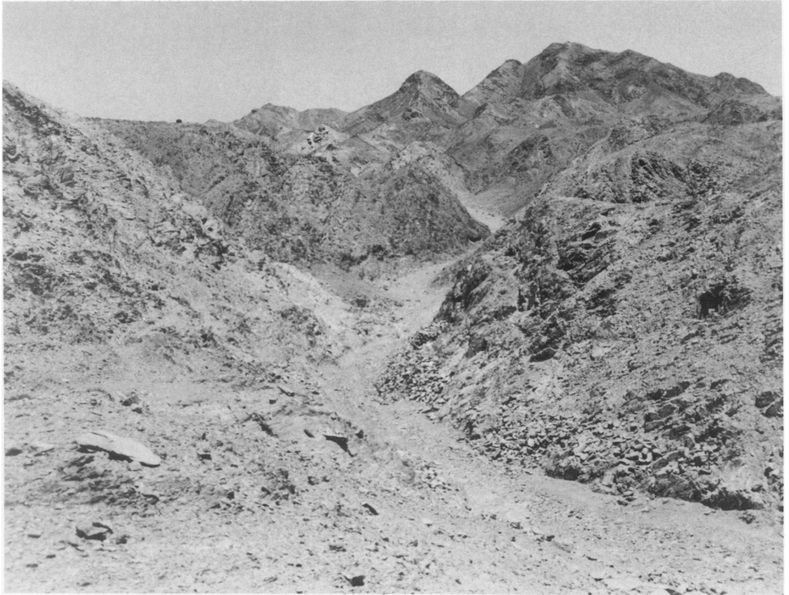
1. The steep and narrow pass across the east-west watershed. The stone retaining walls are evident at frequent intervals (p. 161)
