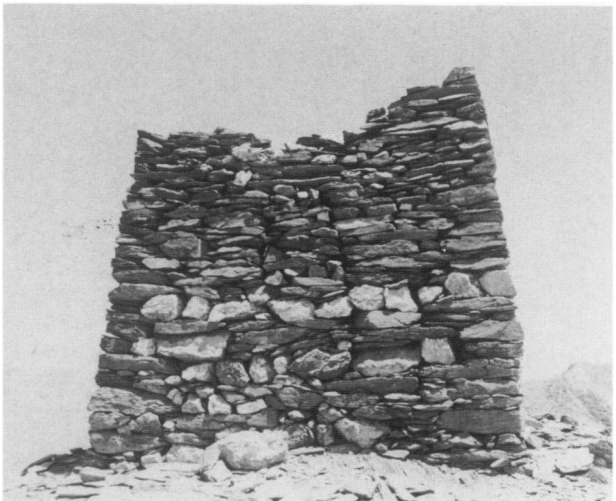
4. Tower in the el-Fawakhir district showing a previously constructed 'window' that is now filled in (p. 182)
